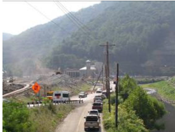
Location #2 – Looking east from the Corps Bridge
