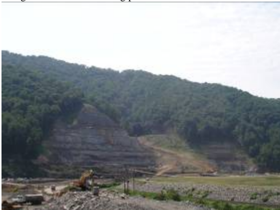
Route 460 Cut Section
