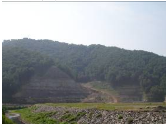
Route 460 & Route 460 Temporary Connector Cut Sections
