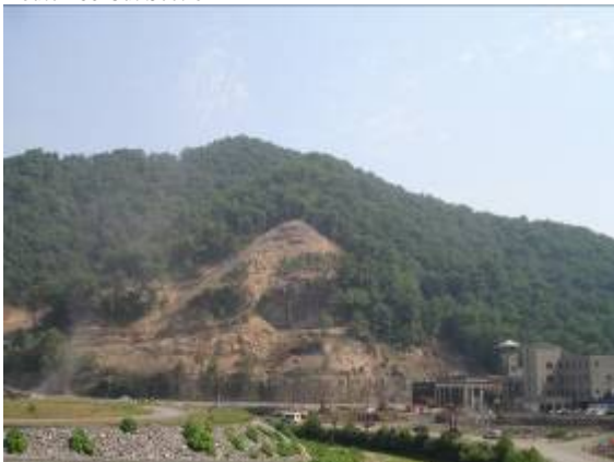
Route 83 Cut Section
