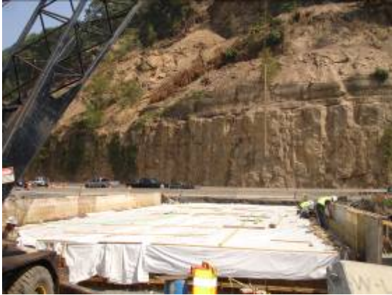
Bridge B627 Deck following placement
