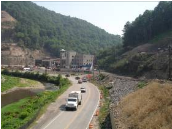
Location #3 – Looking west from Railroad Avenue Bridge
